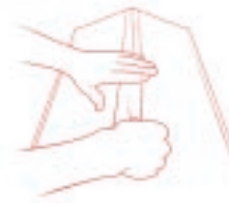
Stand the joined panels with the foil side in to apply the last strip of tape to the outside.
