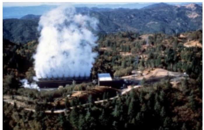
A geothermal heat utility.
