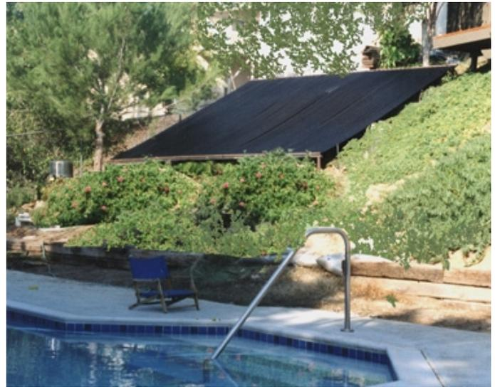
The black panels near the pool side are metallic heat exchangers that absorb solar energy efficiently, and use this cost-saving energy to heat the pool.
