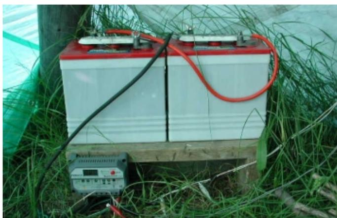
This battery is designed for use with a photovoltaic system, and can be discharged and recharged many times.
